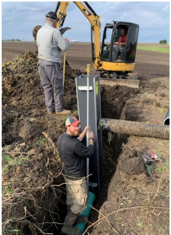
Figure 4. A control structure being installed in the treatment watershed by landowner and research assistant, Jacob Wood (pictured).
