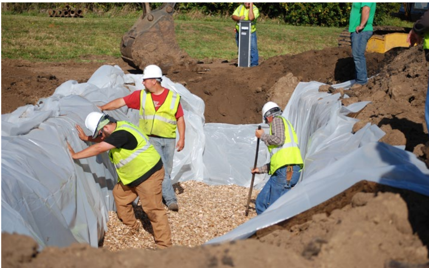
Picture of previous woodchip bioreactor installation.
